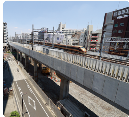
FRP sound insulation wall (bridge railing)
