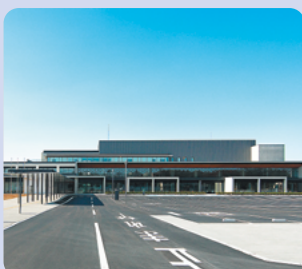
Government building construction (Tobu Construction)
