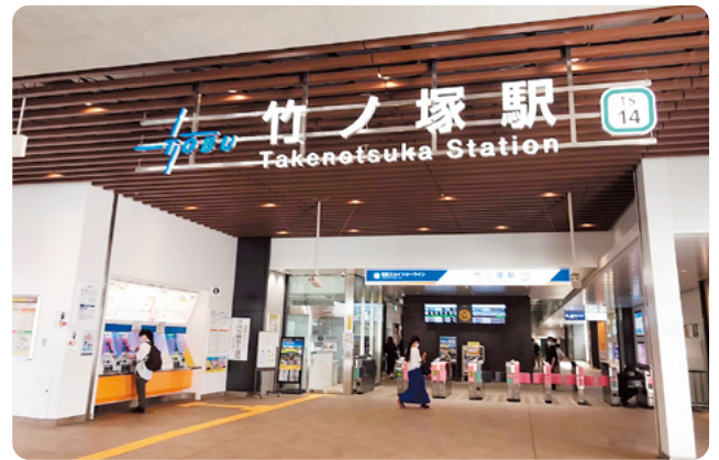
Ceiling lights at ticket gate of Takenotsuka Station
