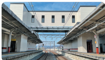
Elevator (Shinkiryu Station)
