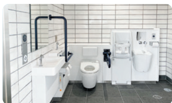
Barrier-free toilet (Omochanomachi Station)
