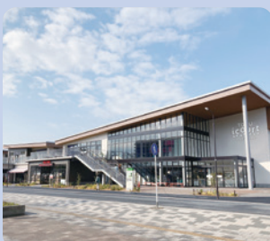
Construction of commercial facilities (TOBU icourt) (Tobu Yachida Construction)
