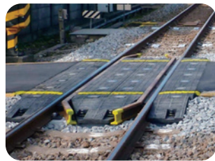
Recycled plastic railroad crossing boards
