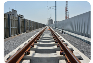
Elastic sleeper bonded directly to the track
