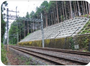
Slope reinforcement
