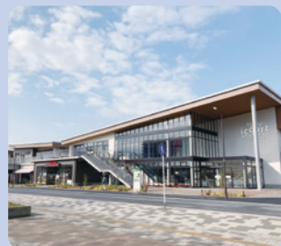
Construction of commercial facilities (TOBU icourt) (Tobu Yachida Construction)
