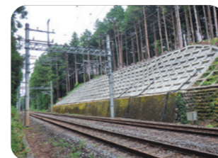
Slope reinforcement
