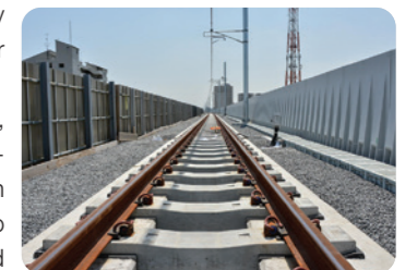
Elastic sleeper bonded directly to the track
