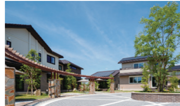
BRIDGE LIFE Platform Minami-Kurihashi
