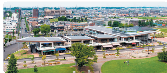
"TOBU icourt" Commercial Facility (Soka-shi, Saitama)
