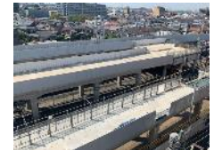
Elevation project in area around Takenotsuka Station
