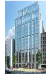
AC Hotels by Marriott Tokyo Ginza construction
