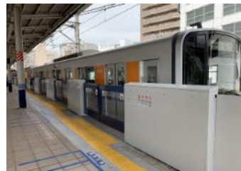
Shiki Station platform door
