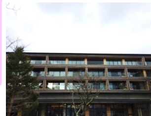
THE RITZ CARLTON NIKKO construction
