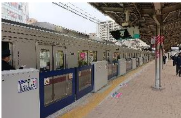
Asaka Station platform door
