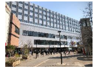
Wakoshi South Exit station building construction
