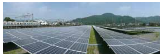
Solar power generation (mega-solar) business
