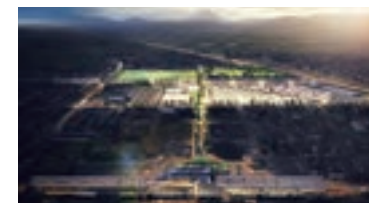
BRIDGE LIFE Platform 南栗橋
