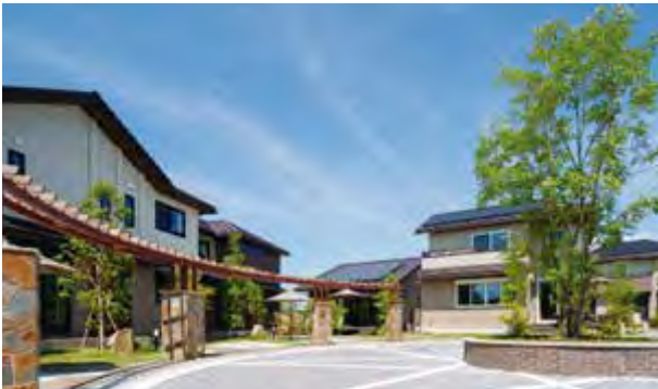
BRIDGE LIFE Platform南栗橋
