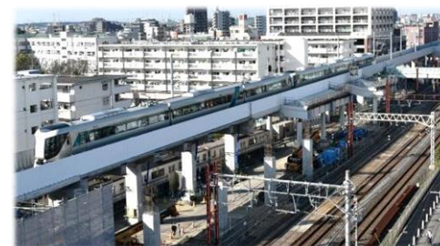
Construction in area around Takenotsuka Station
