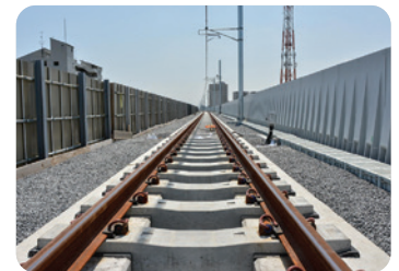
Elastic sleeper bonded directly to the track
