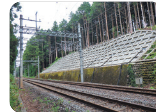
Slope reinforcement
