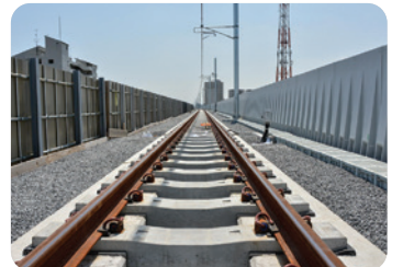
Elastic sleeper bonded directly to the track
