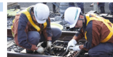
Employees inspecting a railway switch
