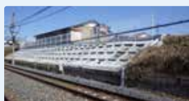
Slope repairs (between Fujioka and Shizuwa)
