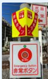
Railroad crossing obstruction alarm device (button type)
