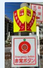
Railroad crossing obstruction alarm device (button type)
