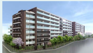
Solaie Katsushika-Kosuge (completed in FY2018)
