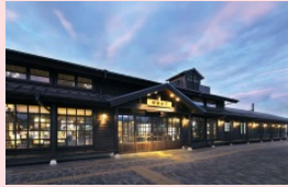
Shimo-imaichi Station building renovation
