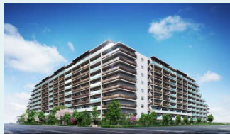
Solaie Nagareyama-otakanomori (completed in FY2019)
