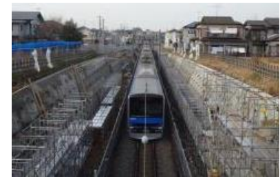
Construction of double-track line between Mutsumi and Sakasai
