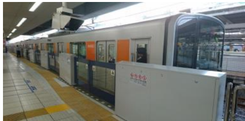
Ikebukuro Station platform door
